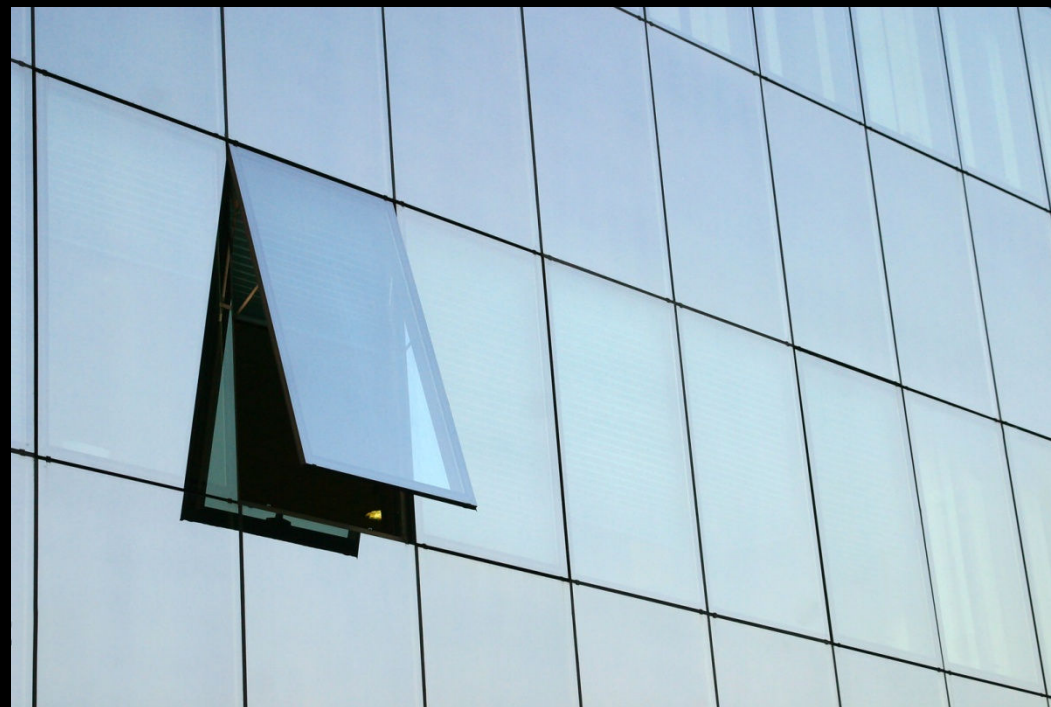
EXAMPLE: OPENABLE FAÇADE PANELS
